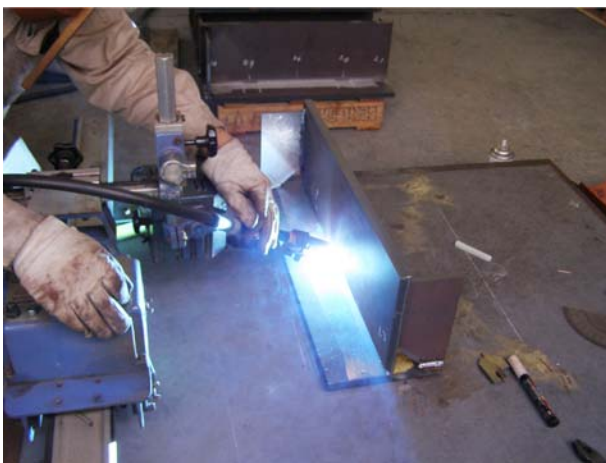
Fig. 2 Picture of full penetration welding method of T joints using high current pulsed MAG welding.
